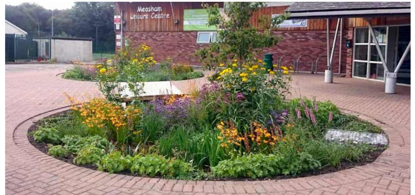
Two shallow raingardens provide storage at Measham Leisure Centre. Robust ground cover should persist through winter in order to protect soils.
