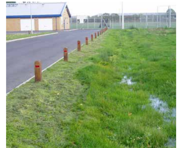
Pershore High School, Worcestershire. Low risk access road with 1.2m wide filter strip source control and conveyance swale.
