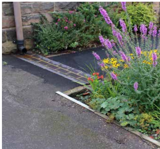
Strutts Centre, Belper. A retrofit downpipe shoe and brick channel into a raingarden.
