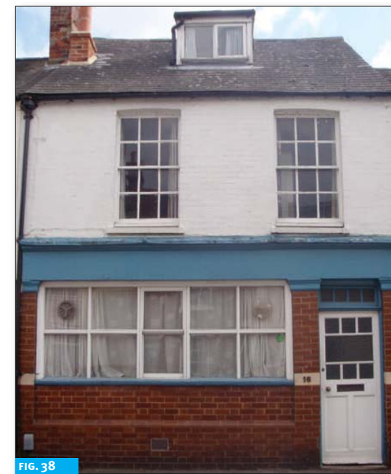
FIG. 38 Former shop front, Bridge Street
