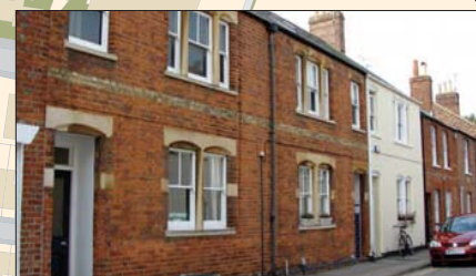
West Street Characterised by terraced housing of various styles including some of the earliest houses on the island and two ranges of rubble stone houses
