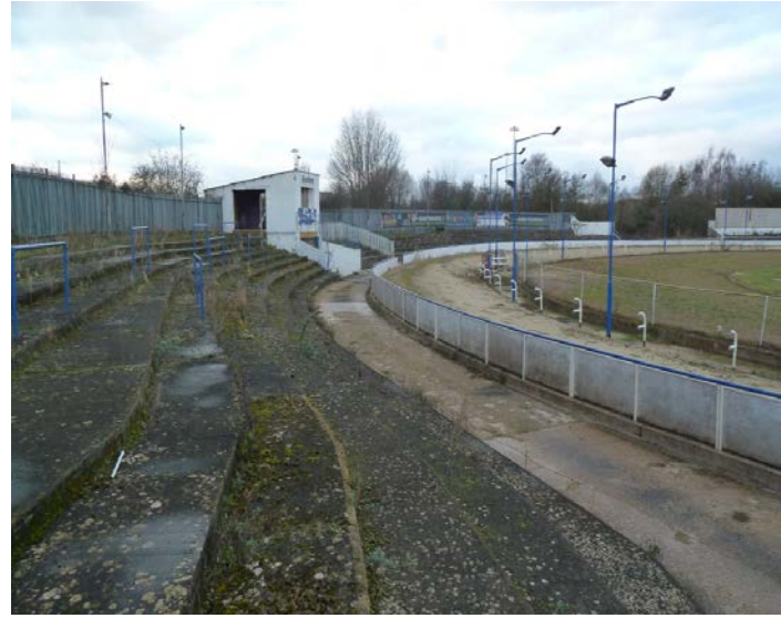
Fig 4: The concrete western terraces (built c 1939) are in many ways exemplary of their time both in their design and materiality (i.e. form). Their location in quite close proximity to the dog tracks catered to the 'modern desires' of their audiences who increasingly sought more heightened sensorial stimulation through greater contact with the 'main action'. Their curving design following the general line of the track enable spectators to view the unfolding of a race from start to finish without the need for binoculars as was often the case with other sports such as horse racing. Their material construction - consisting primarily of large expanses of moulded concrete - embody the modernist movement's preoccupation with ephemeral as well as catering to the need for expedience that was generally necessitated in the construction of pleasure buildings.
