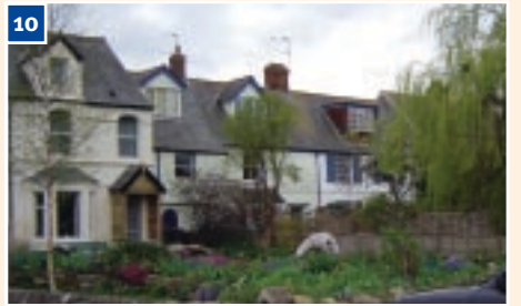
10 'Back to Front' Houses, Godstow Road these houses are thought to have originally overlooked Wolvercote Common with the Godstow Road frontages being the rear elevations
