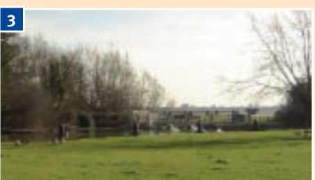
3 Godstow Lock Originally constructed in 1790 following the building of the canal. Present concrete structure was constructed in 1924 and was the last lock on the Thames to be mechanised.
