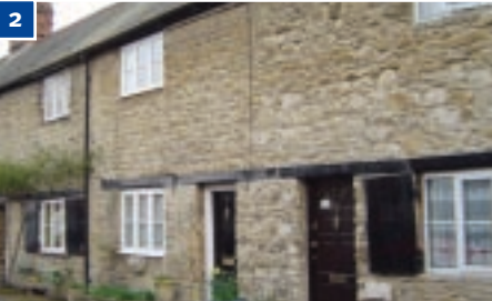
2 Mill Road Cottages Grade II dating from late 18th century constructed from coursed rubble stone with slate roofs
