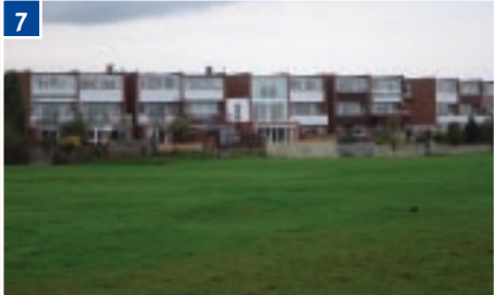
7 Rowland Close 20th century development outside the conservation area having a negative impact on the character of the area
