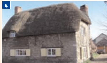
4 Nunnery Close Grade II, the oldest house in Lower Wolvercote dating from the 17th century. Coursed rubble stone with thatched roof
