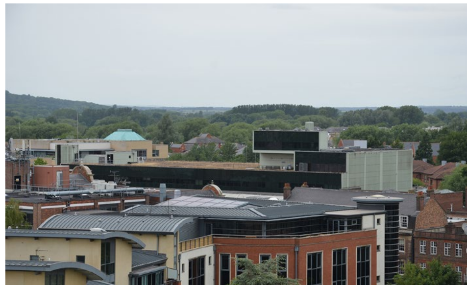
Beaver House - long flat rooves detract from the skyline (OCC)
