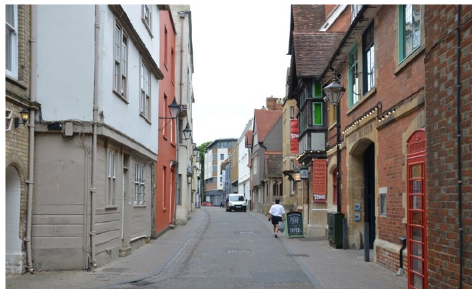
Pembroke Street - facades have been retained but the loss of their original use is to the detriment of the vitality of the street (OCC)
