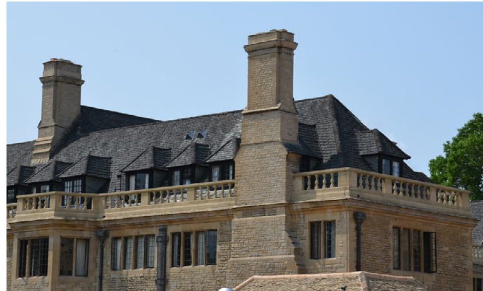
Rhodes House - coursed rubble stone with Clipsham dressings and slate roof (OCC)
