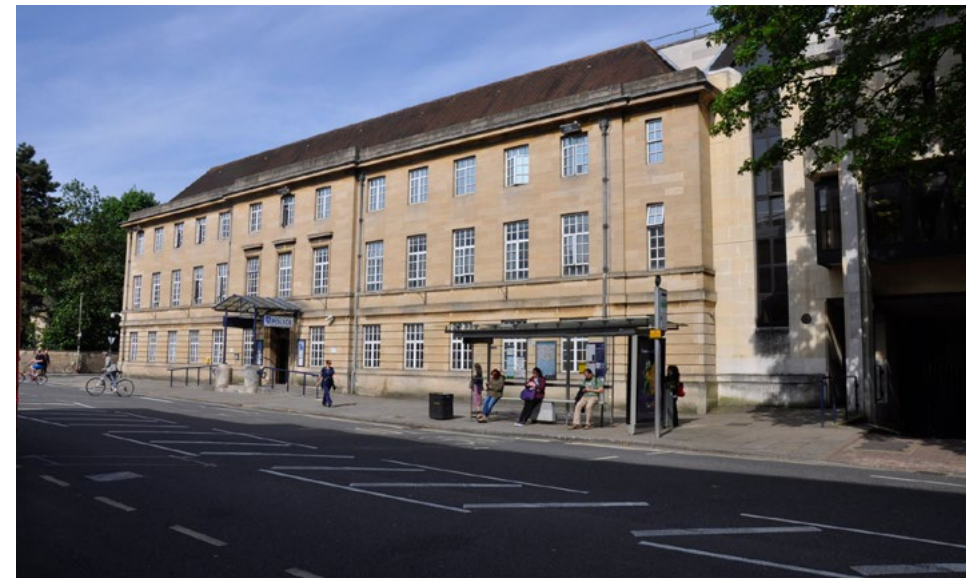
Oxford Police Station (1936) by H.F. Hurcombe, the City Estates surveyor, faces onto St. Aldates.
