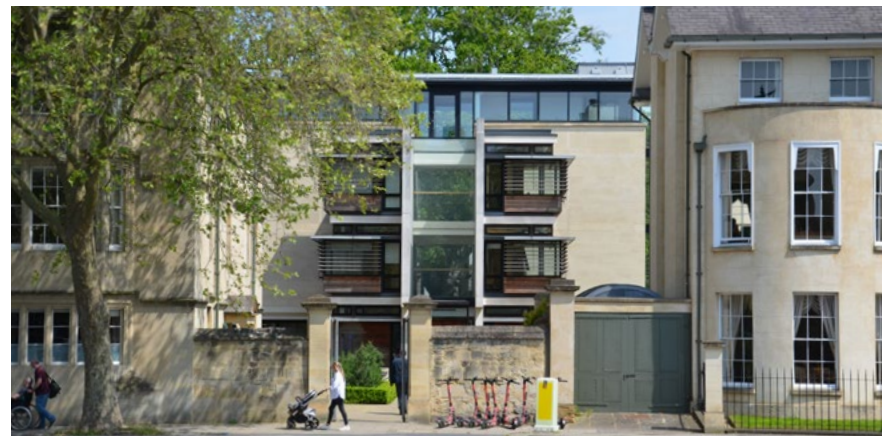
St John College Kendrew Quad by MJP - relates well to its context (OCC)
