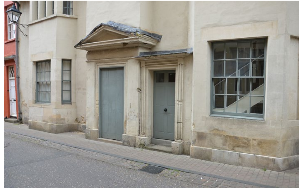
Original windows no longer serve habitable rooms (OCC)
