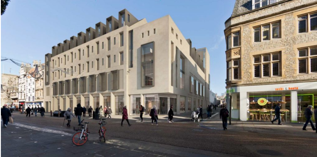
Image 1: Northgate House upon completion
