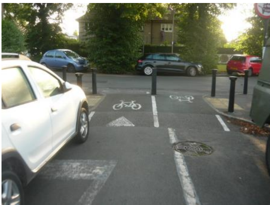
Figure 52. Traffic filter in Freelands Road
