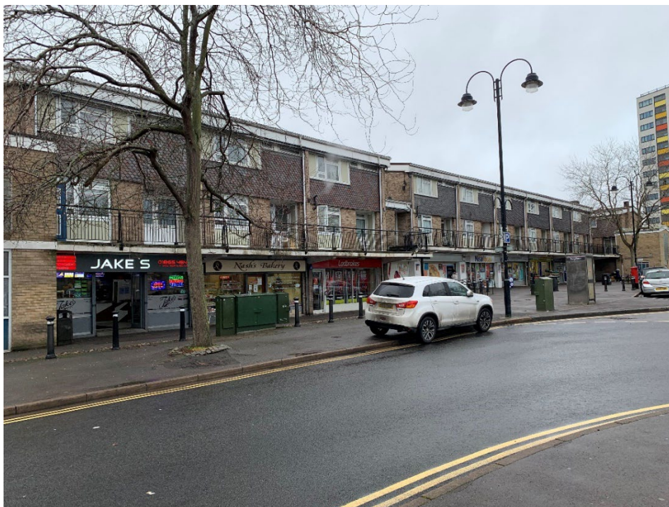
Figure 4-26 Parade of shops along Blackbird Leys Road ('Top Shops')
