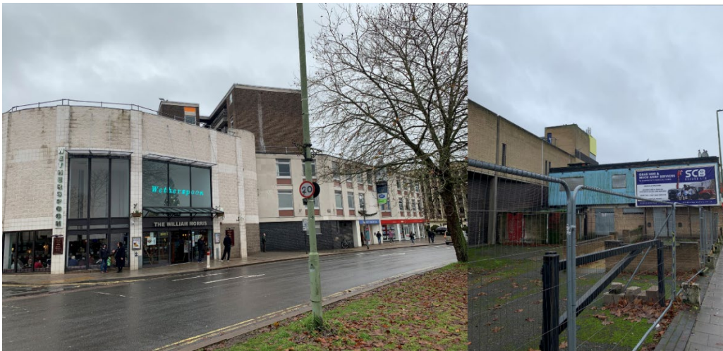
Figure 4-12 Exterior of shopping centres and temporary fence panels
