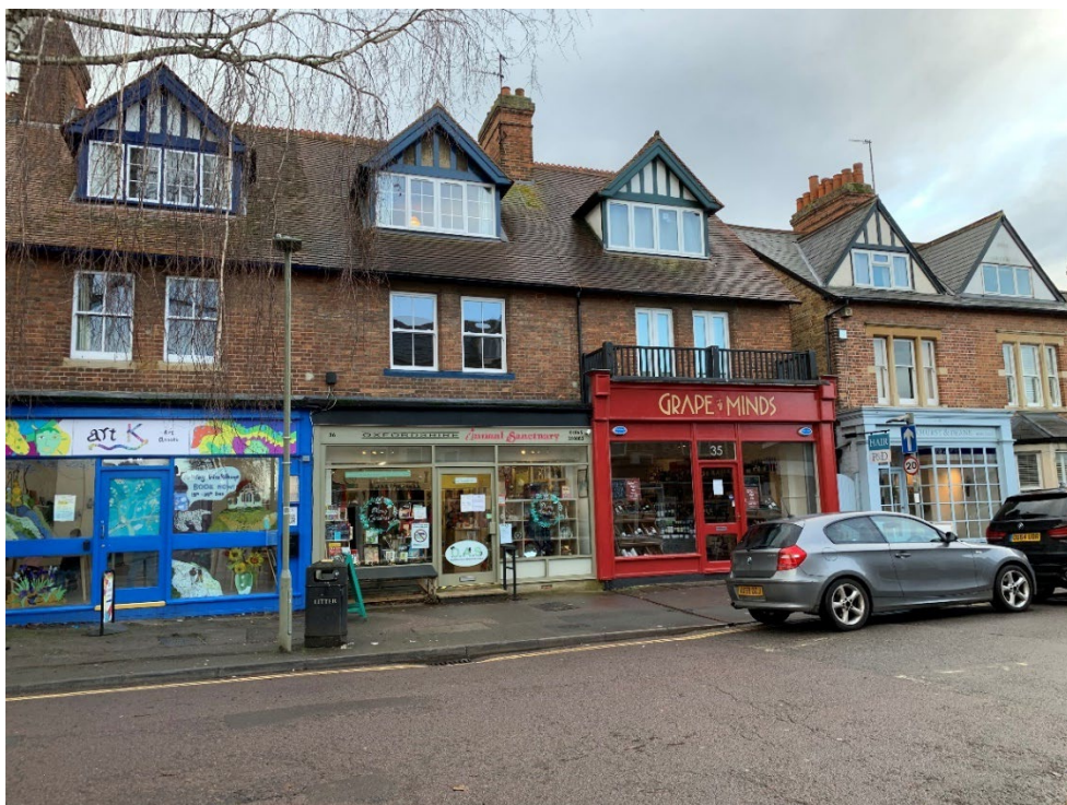
Figure 4-20 Attractive façades along South Parade
