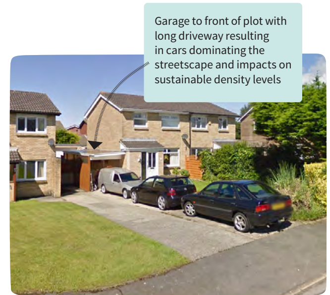
Typical inefficient 80s parking solution
