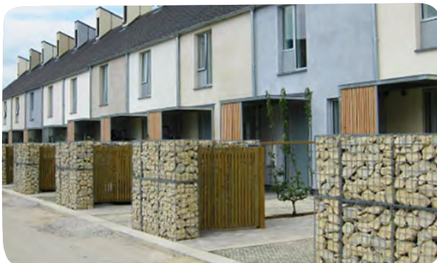
Bin stores designed into the front of homes
