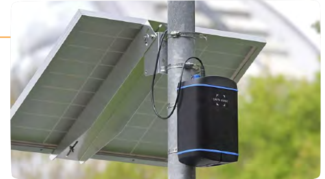
Street light with mounted air quality sensor.
