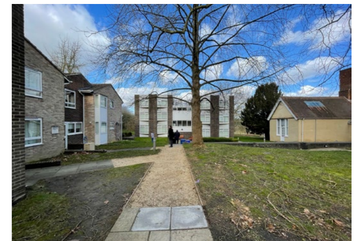
Existing western campus and accommodation blocks
