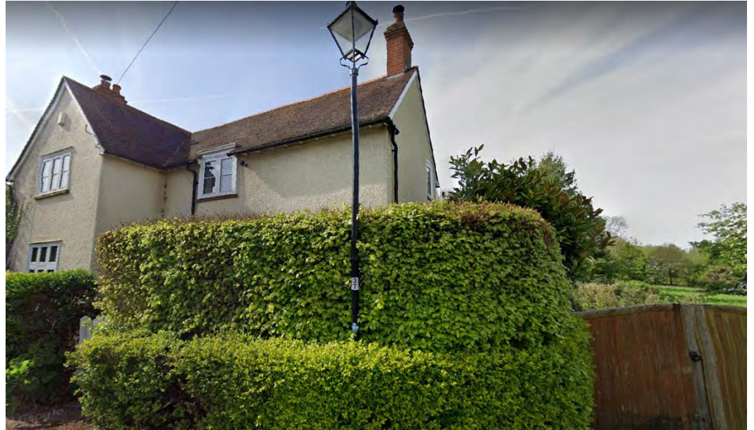
Plate 11 400 Meadow Lane viewed from Meadow Lane with the subject site to the right of the image (source : Google Street View)
