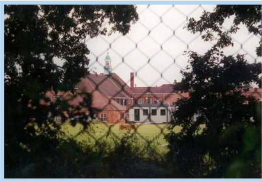
Photo 1: Headington Girls School, a neo-Georgian building was added in 1928.
