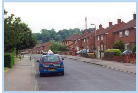
Photo 2: More recent brick housing with development on one side of the street only.
