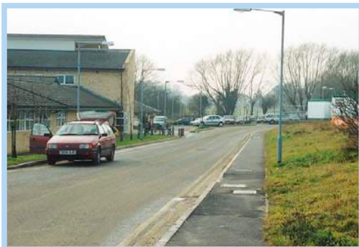
Photo 3: The hospital access road has concrete kerbs and municipal lights.
