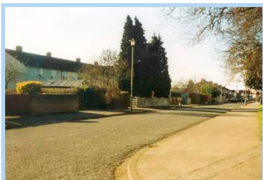
Photo 5: Back garden fences exposed to the public realm.
