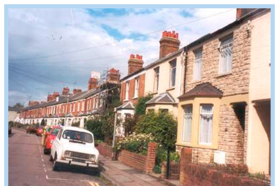
Photo 6: Low red brick walls, fenestration and doorways unite the streetscape.
