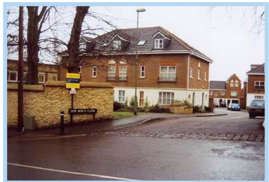
Photo 4: New cul de sac development has created a new townscape pattern.
