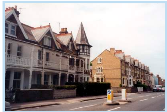
Photo 4: Distinctive buildings with turrets and balconies on the Abingdon Road.
