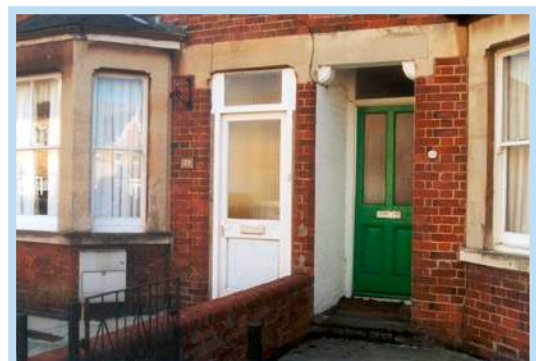
Photo 6: Incremental changes in doorways and fenestration alter the character of the streetscape.
