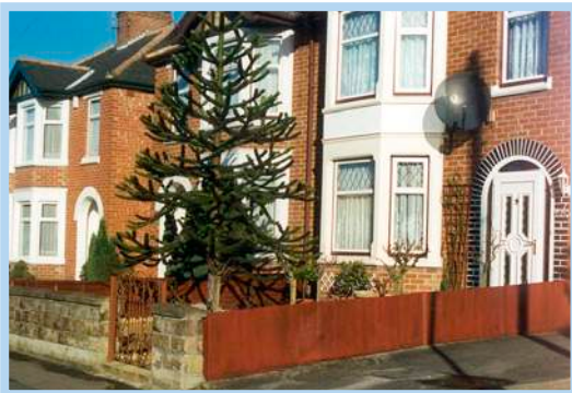
Photo 3: Home improvements - new windows, door and other features.
