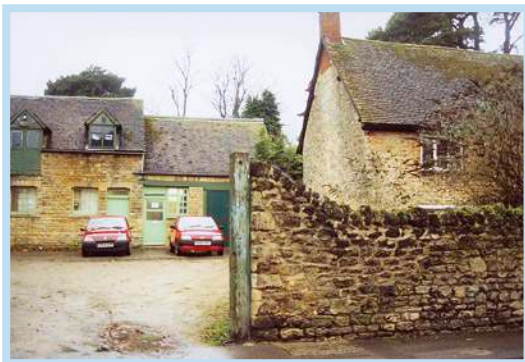
Photo 3: Historic walls and buildings.
