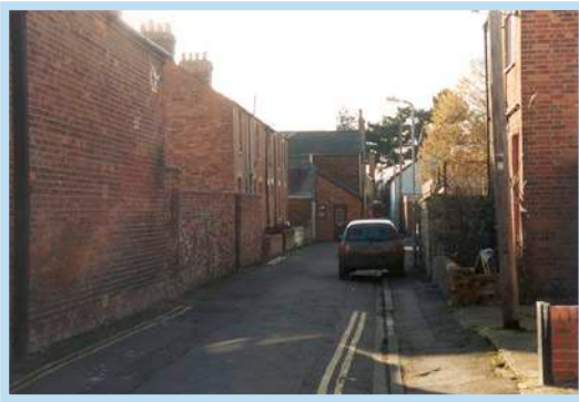
Photo 1: Doors lead directly onto the street.
