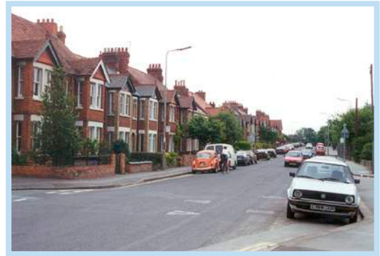
Photo 2: Later Victorian and Edwardian houses have gables to the front and two storey bays.
