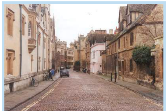
Photo 4: High density of architecturally distinctive buildings contribute to townscape quality.
