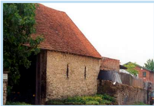
Photo 3: Rural agricultural buildings in the village core.
