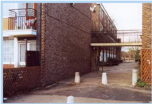
Photo 7: Approaches to river through new housing area off Thames Street.
