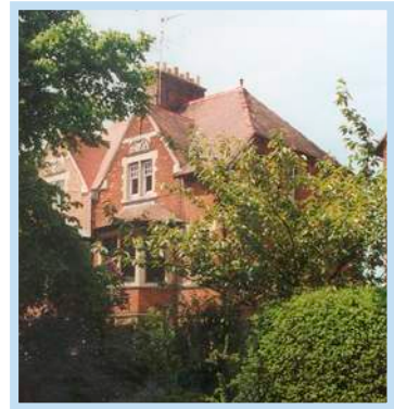
Photo 2: Buff red brick detailing and gothic architecture is typical.
