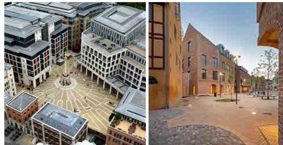
Providing a sense of enclosure to a space that is proportional to its surroundings is a key principle
