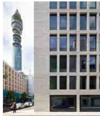
Softening large buildings with active frontages and façades broken up by windows
