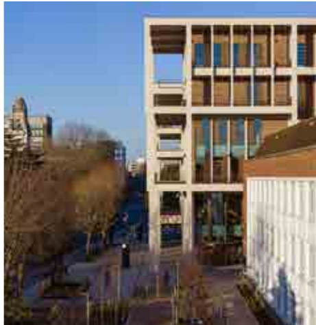
Architecture and public realm which creates a destination and gateway into Oxford
