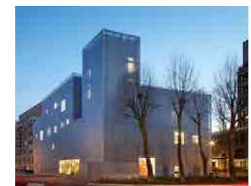
Marker buildings could be bespoke single use buildings, such as this Energy Hub, whilst also aiding wayfinding
