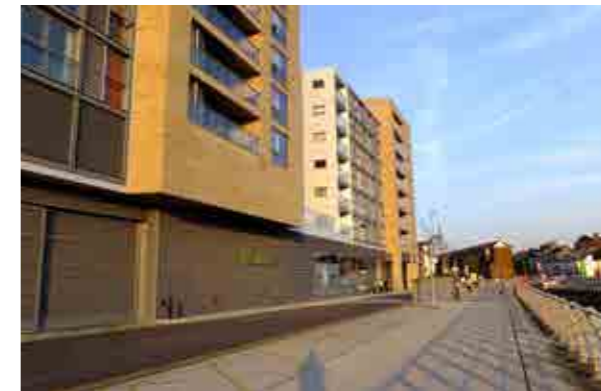
This retail unit presents a blank façade at ground level
