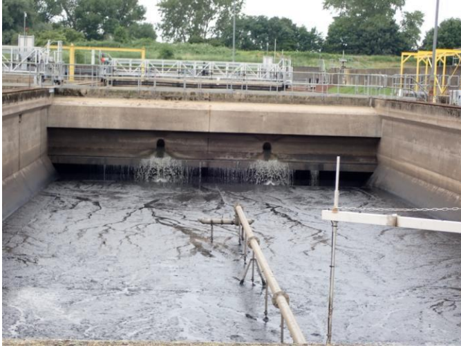
Photograph 3 - Sludge in Storm Tank 2
