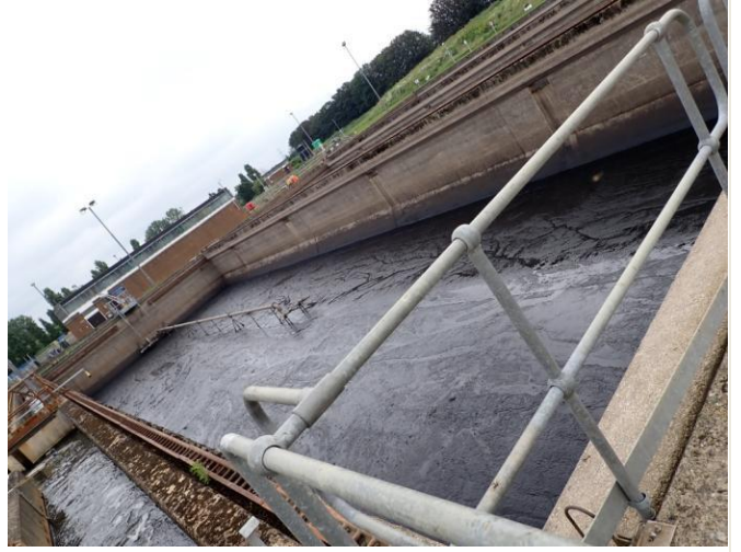
Photograph 4 - Sludge in Storm Tank 3
