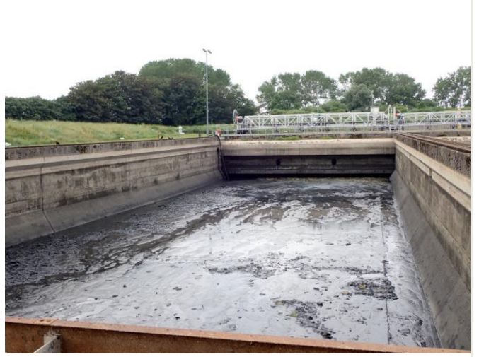
Photograph 4 - Sludge in Storm Tank 3
