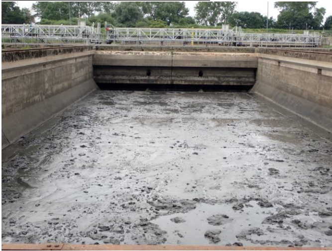
Photograph 5 - Dark septic sewage being held up between storm overflow and Storm Tank 3
