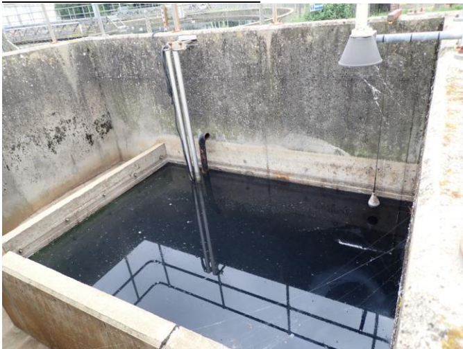
Photograph 5 - Dark septic sewage being held up between storm overflow and Storm Tank 3
