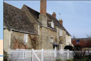
Bartlemas Farmhouse 14 th and 15 th century core with 17 th , 18 th and 19 th century additions predominantly constructed from rubble stone.
