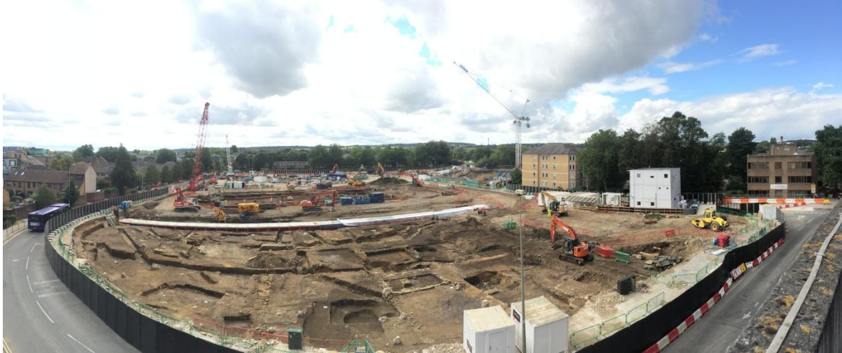
Westgate Area 7: showing buildings belonging to the Franciscan Friary (Picture by Oxford Archaeology).
