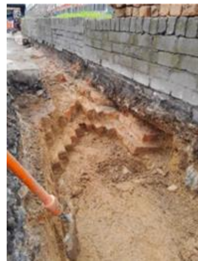
Image above left: Network railing illustration of the inverted brick arch. Image right: Part of the unusual inverted brick arch at Botley Road (Images courtesy of Network Rail).
