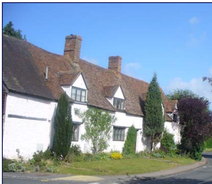
The long, low frontage of Cross Farmhouse
