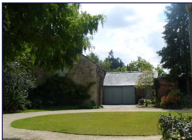
Former farmyard at the rear of Alan Court including a small barn
