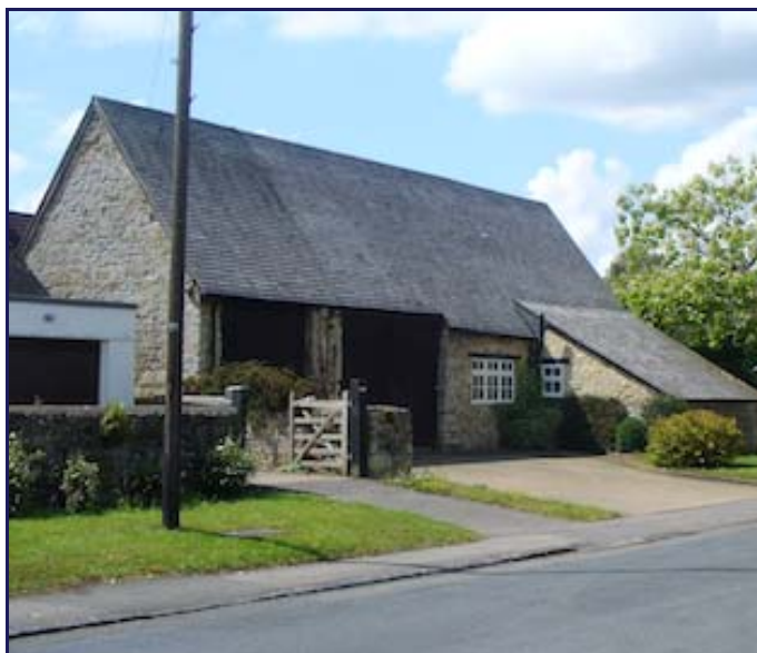
Converted barn at No. 4 Elsfield Road
