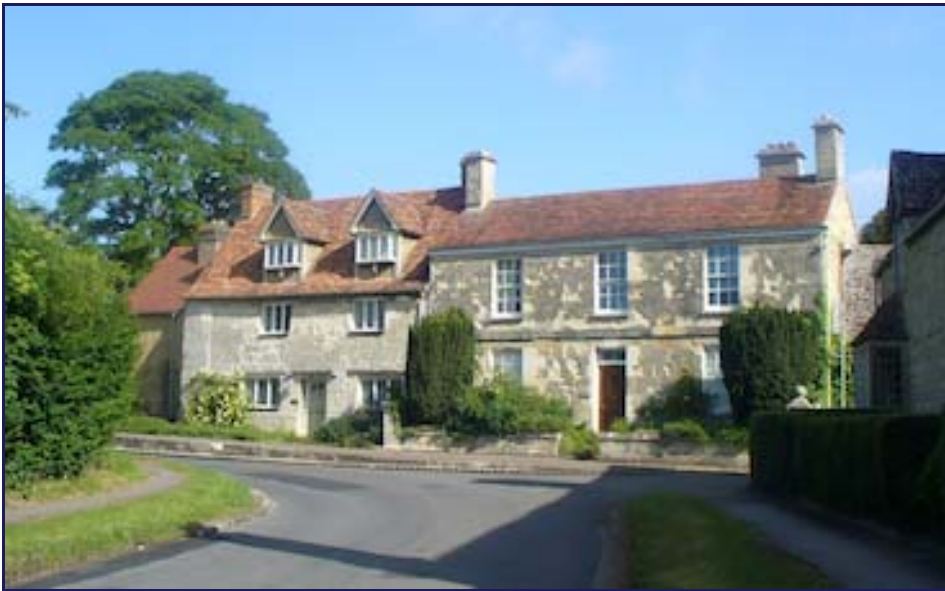
Cromwells House and The Manor (Nos. 17 and 15 Mill Lane
