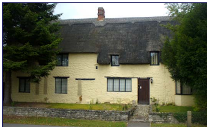
Fir Tree Cottage, converted from two limestone rubble cottages with a thatch roof including a later 20 th century style 'block ridge'
