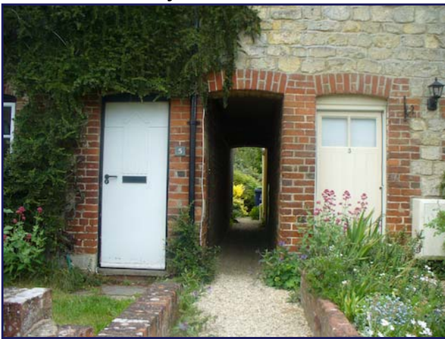
Cottage doorways outlined in brick at Mill Lane.
