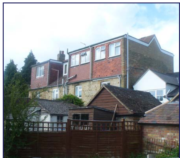
View of the rears of Oxford Road cottages from Boulds Lane
