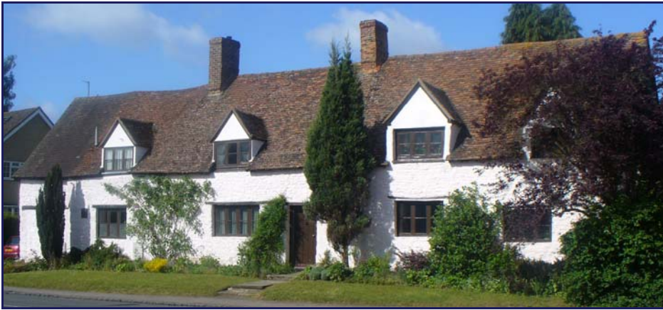
Cross Farmhouse exemplifies the steeply pitched roof of local hand made tile, dormers rising flush with the wall, retention of timber lintels over casement windows and other features of the area's local vernacular style
