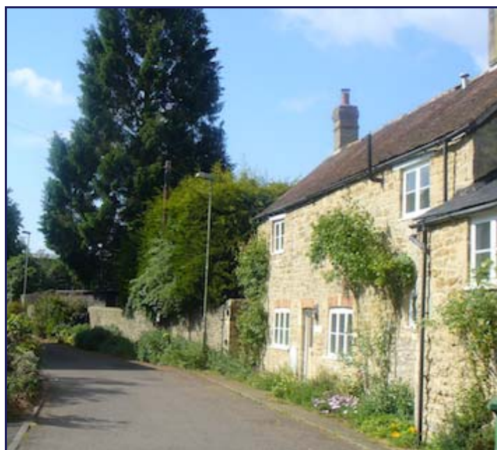
Church Farmhouse, Church Lane (north)
