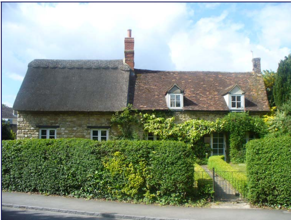
No. 38 Oxford Road, partially rebuilt, provides many of the distinctive features of the local vernacular cottages
