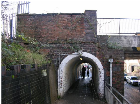
Botley Road railway bridge looking west
