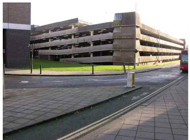
Westgate Car Park designed by the City Architects Department (looking south).
