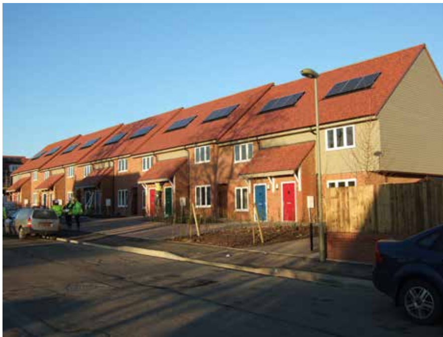
Solar panels on new council housing on Lambourne Road
